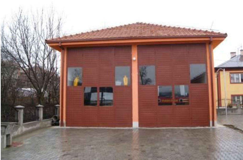
Construction of a garage for two fire vehicles
