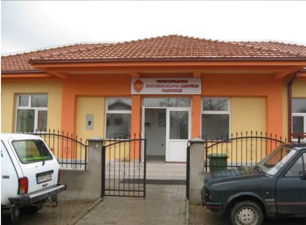
Reconstruction of a facility fire house
