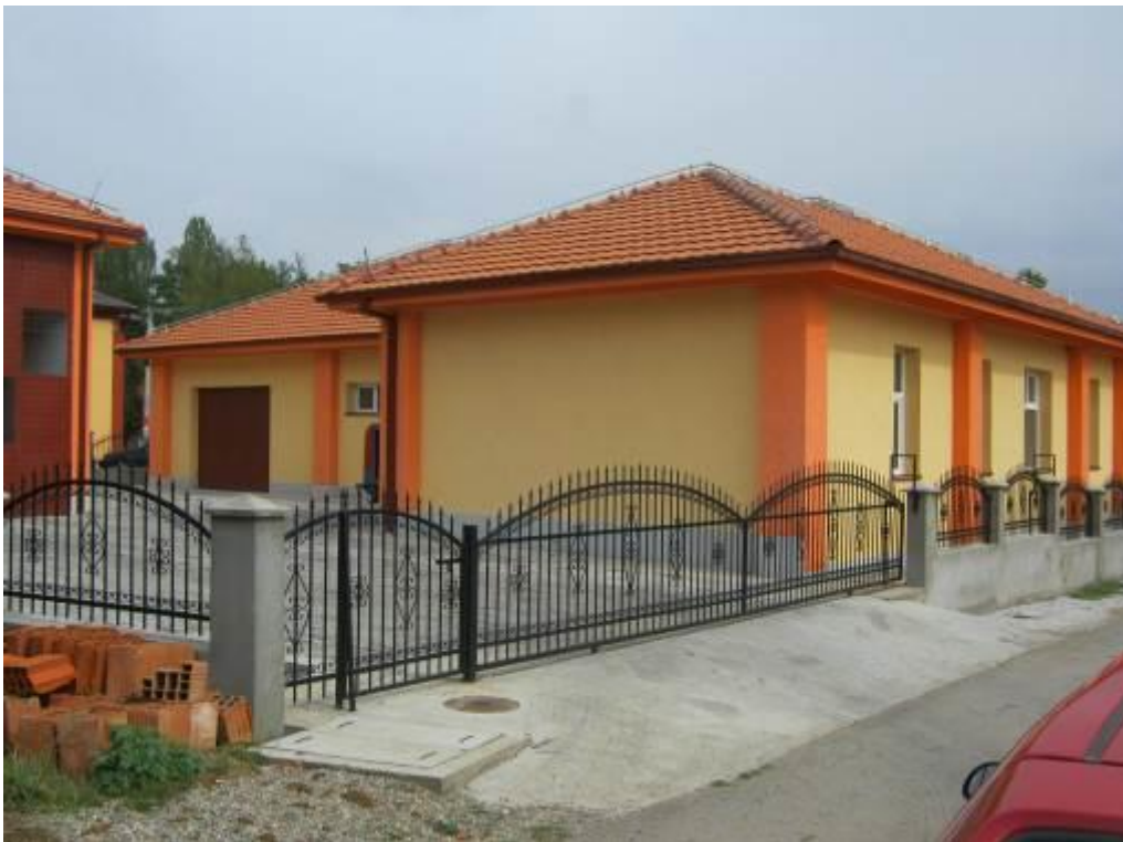
Fencing and landscaping the yard around the building
